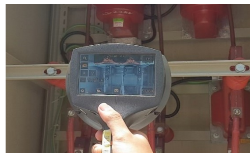
Fig 1. Acoustic partial discharge detector named NL camera.
