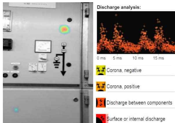
Fig 14. Surface/internal discharge detected at 3.3 kV switchgear.
