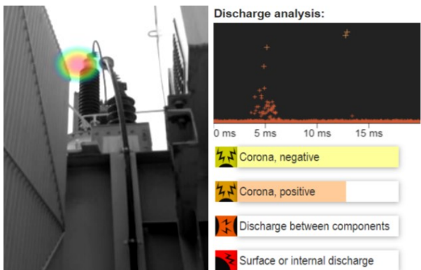
Fig. 11. Positive corona discharge at 115/24 kV bushing of transformer.
