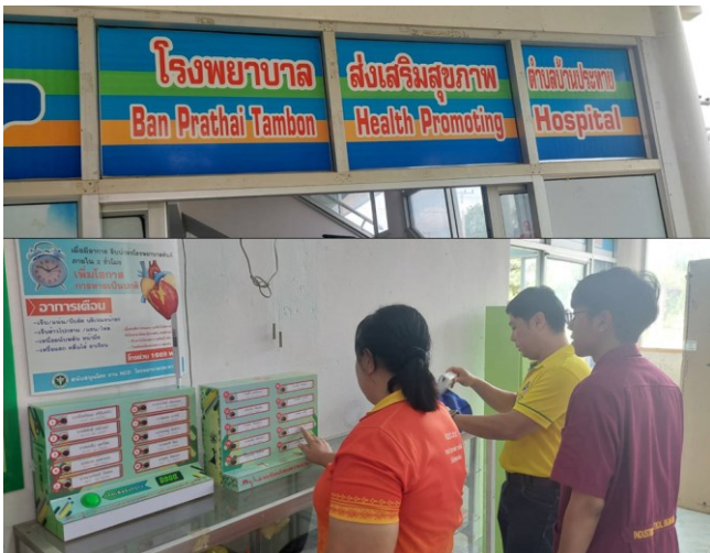
Fig. 14. Receiver equipment installation.
