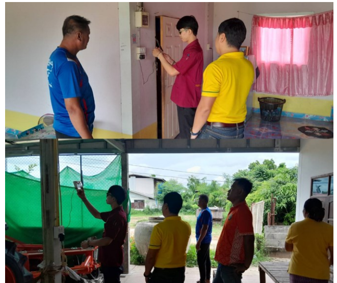
Fig. 15. Transmitter equipment installation.
