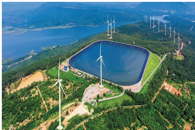
Fig. 4. Wind Turbines Phase 1 & 2 Project around Lam Takong Reservoir
